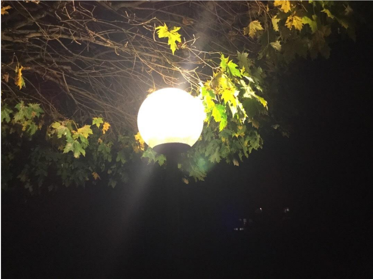
Fig.16 Globe lights in a housing development. Needs shielding to prevent upward emissions.
