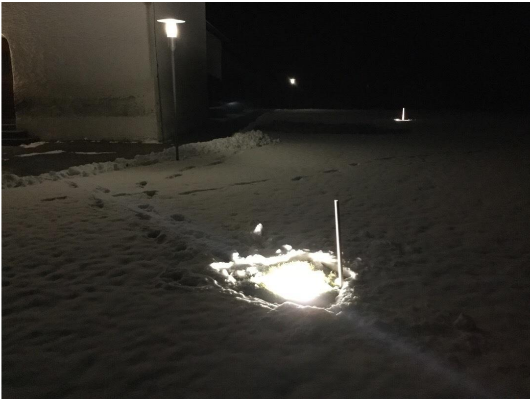
Fig.18 Ground based floodlight – should be replaced with structural down-lighting.
