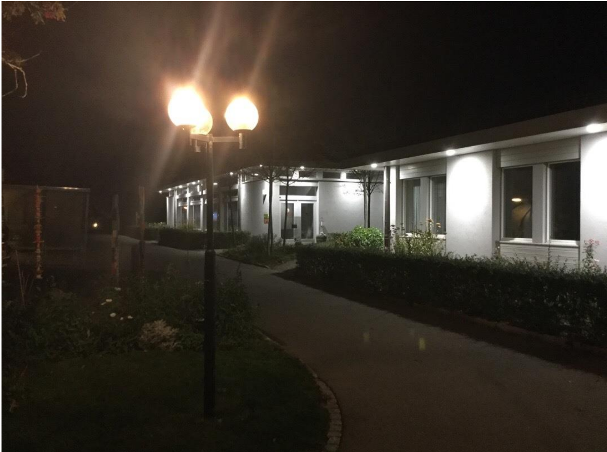
Fig.15 Globe lights in a Wohnheim/Pflegeheim – 50% of lighting is of no use, being emitted upwards to cause skyglow. Possibility to retrofit „hats“ to block upward emissions.
