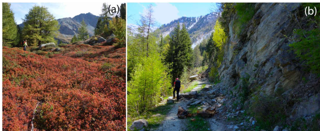
Figure 3. (a) Closed elongated depression at the top of the Böchtur hillslope, possibly indicating a Sackung-type failure of the bedrock, (b) local slope collapses near the bend of the road described in the text. Photos by B. McArdell, WSL.
