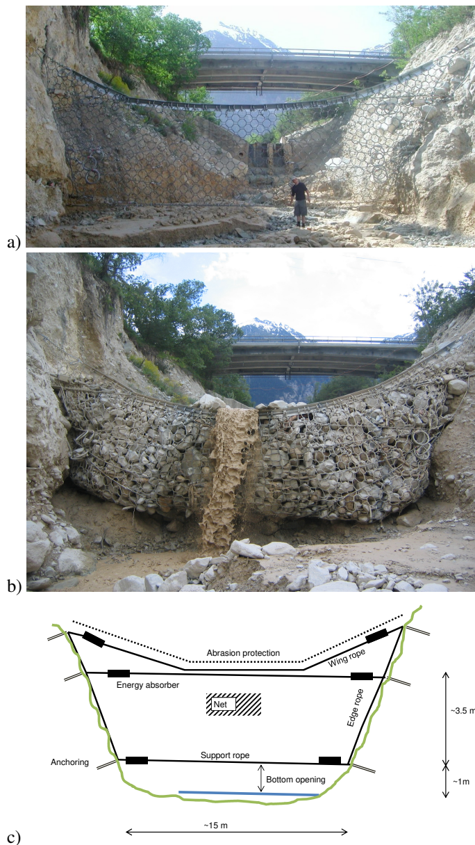
Fig. 1. a) Flexible debris flow barrier in Illgraben torrent (Switzerland; b) Flexible debris flow barrier in Illgraben torrent (Switzerland after debris flow event from 18 May 2006; c) possible arrangement of structural components of a flexible debris flow barrier (Volkwein, 2014) and its rough dimensions in Illgraben torrent.
