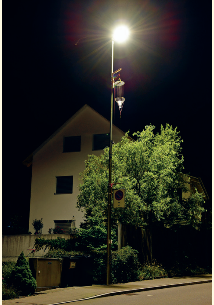
Insect trap mounted on an automatically dimmable LED street lamp.
