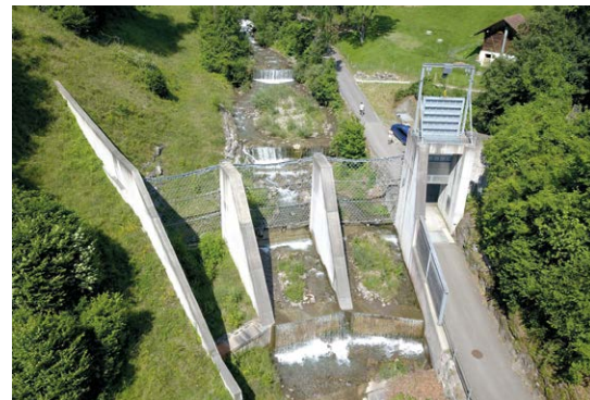
Barrier, downstream side (Image: [F]).
