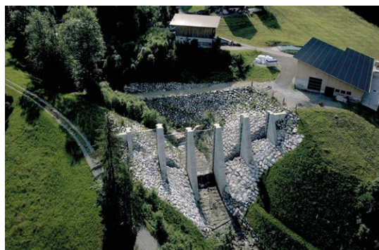
Barrier, downstream side (Image: [F]).
