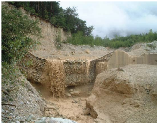
Filled VX barrier for restoration stage 1 (Image: [G]).
