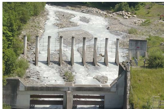
Barrier, downstream side (Image: [F]).
