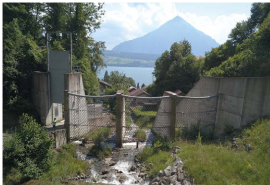
Barrier, upstream side (Image: [F]).
