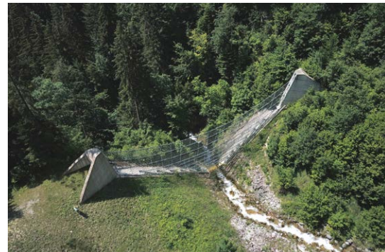
Barrier, downstream side (Image: [F]).
