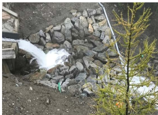
Pre-filled barrier using large blocks, seen from above (Image: [I]).
