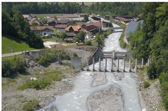
Barrier, upstream side (Image: [F]).
