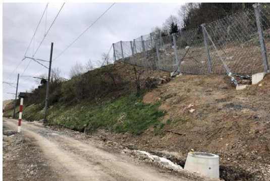
Barrier, seen from below (Image: [H]).
