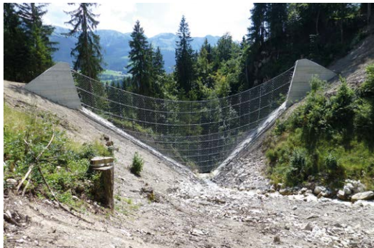
Barrier, upstream side (Image: [F]).
