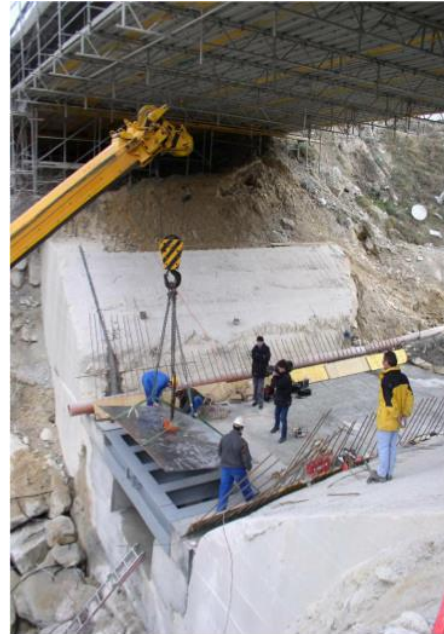
Fig. 2 Installation of the force plate.
