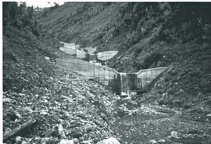
Figure 47. Serie of check dams for channel stabilization [15]
