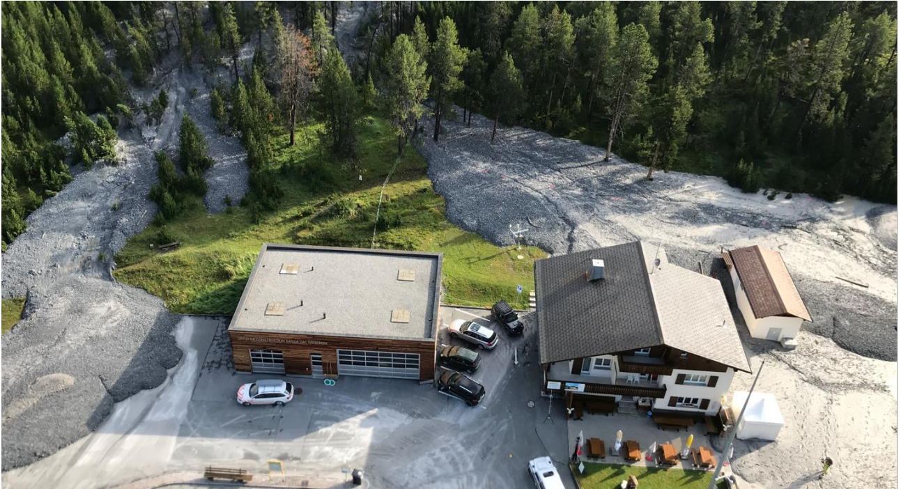
Figure 1.1: Depositions of the debris flow event at Buffalora, reaching the Werkhof and Berggasthaus Buffalora, right at the Ofenpass road. Data: Herzog Ingenieure AG (2022), Herzog Ingenieure AG provided by AWN Südbünden on 2 August 2022, not intended for further use.
