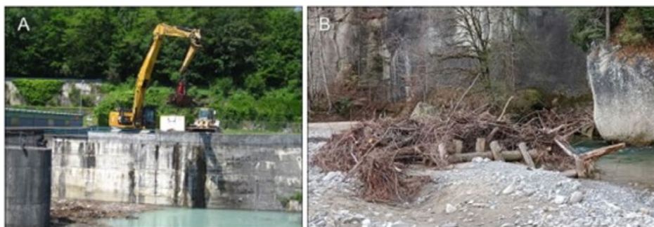
FIGURE 7 | (A) Picture from the Genissiat dam in the Rhone River in France, where the dam managers periodically remove the floating wood from the reservoir. (B) Engineered log jam designed to retain naturally transported wood in the Sense River in Bern (Switzerland). [Color figure can be viewed at wileyonlinelibrary.com ]
