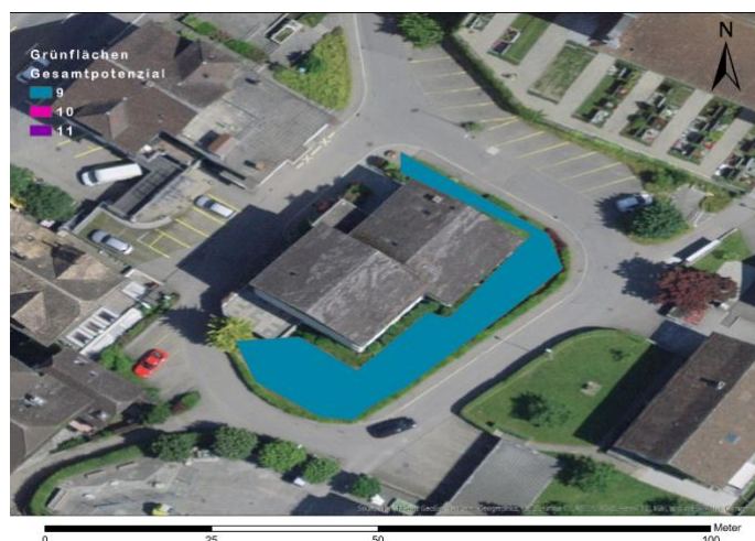
Abbildung 23: Fläche Gemeindeverwaltung. Quelle Hintergrund: Esri, Digital Globe, GeoEye, Earthstar Geographics, CNES/Airbus DS, USDA, USGS, AeroGRID, IGN, and the GIS User Community
