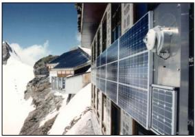
**Fig. 1:** View of the grid connected PV plant (1.1kWp) at the research station at Jungfraujoch (3454m, about 46.5°N): One of the two arrays with irradiance sensor (pyranometer and reference cell).
