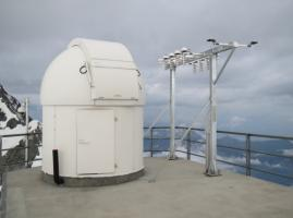
Figure 1. Installation of the new measurement bench on the Sphinx terrace (left) and Jungfraujoch SACRaM station after completion of the renewal. The new measurement bench holds more available positions than the previous one, and all cabling are now located within the metallic structure and are thus protected from the harsh meteorological conditions.
